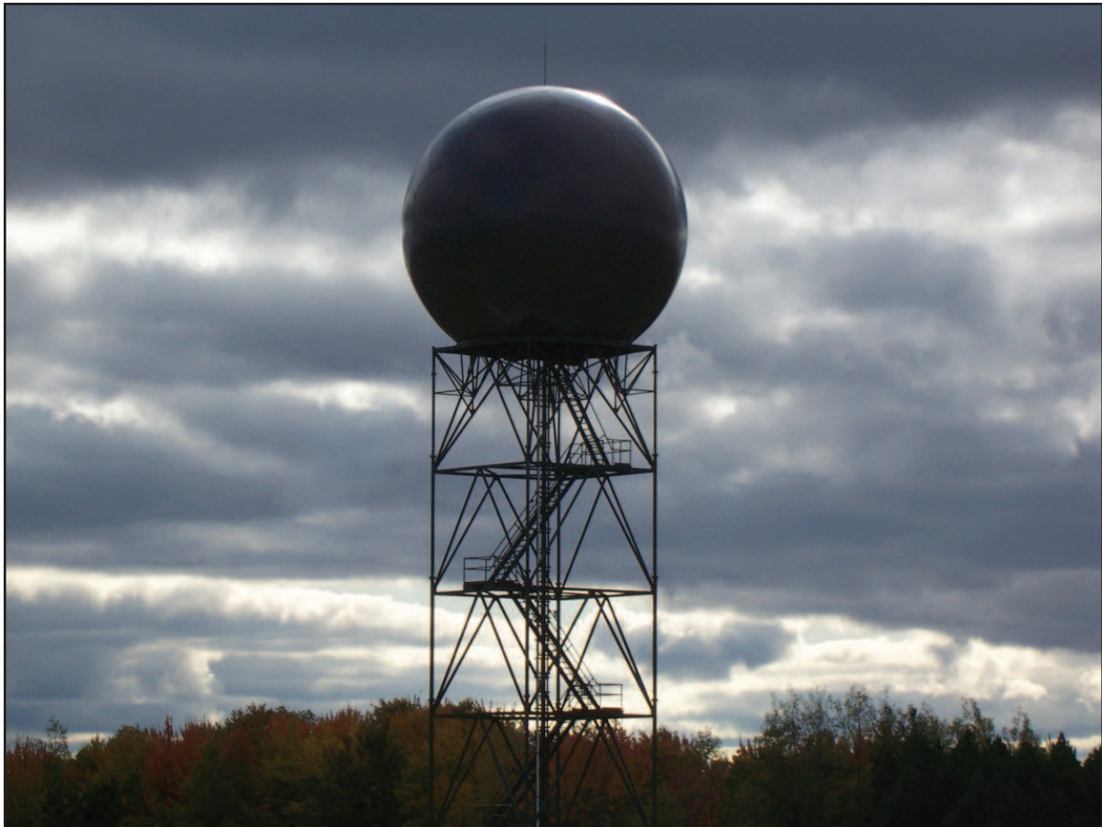
Figure 3. Data from NEXt Generation RADar (NEXRAD, WSR-88D) was used to quantify bird concentrations during migration with direct application to minimizing avian collisions with wind turbines (photo: J. Gehring).
